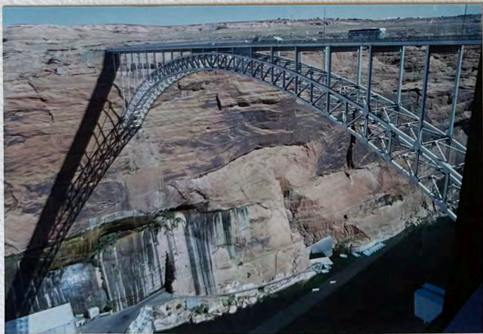
BRIDGE BELOW THE DAM - OVER COLORADO RIVER
